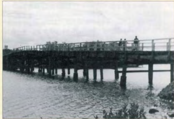
North Creek Bridge
